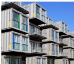
Container / Modulabauten Container/Modular buildings
